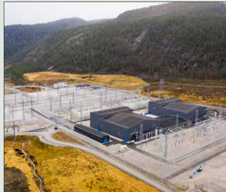
Erstmyra converter station in Norway: the NordLink interconnector links the power grids of Norway and Germany
