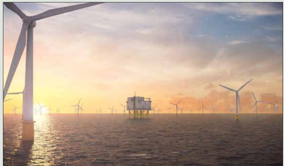
An HVDC platform at the Dogger Bank wind farm. HVDC systems support cross-border energy trading while reliably integrating offshore wind farms. (Photo courtesy of Aibel)
