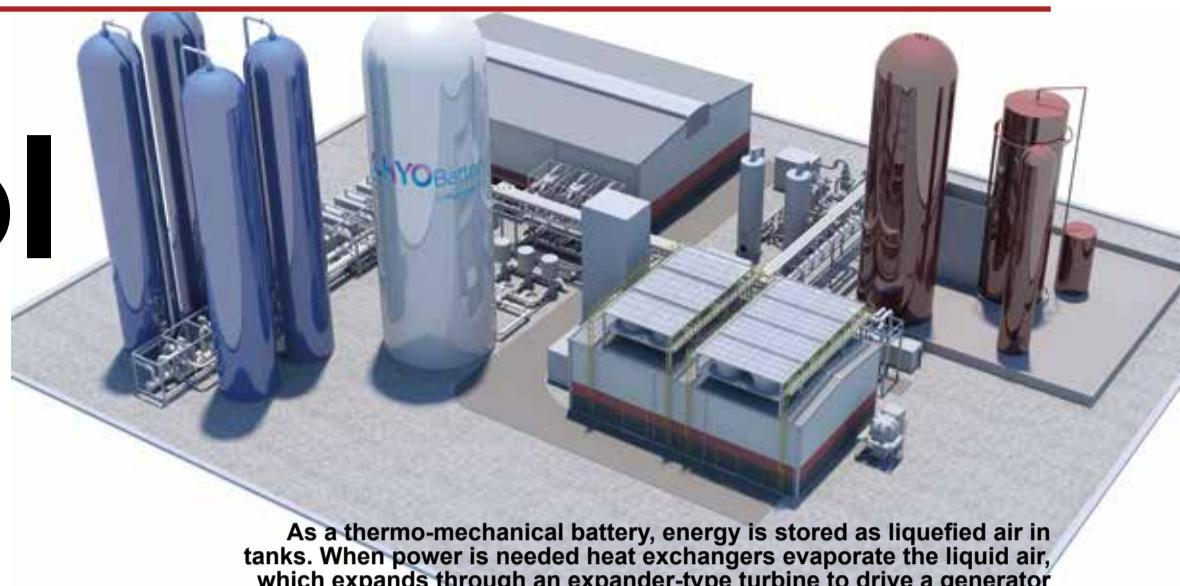
**As a thermo-mechanical battery, energy is stored as liquefied air in tanks. When power is needed heat exchangers evaporate the liquid air, which expands through an expander-type turbine to drive a generator**
