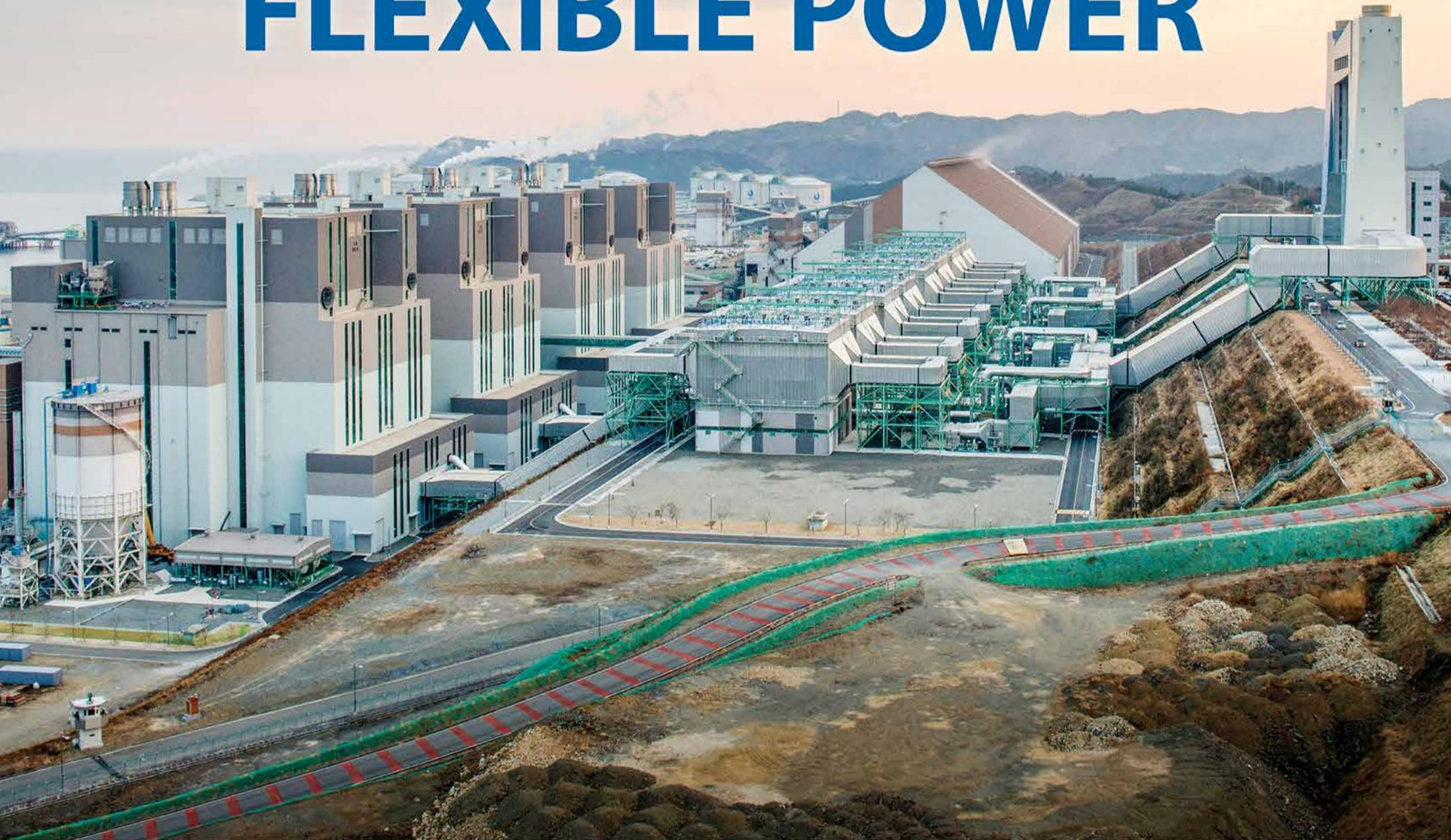
The massive 2.2 GWe Samcheok Green Power Project in South Korea is approaching two years of full commercial operation. Utilizing the most advanced ultra-supercritical CFBs in the world, it signifies the next big step for clean and flexible power from economical solid fuels.
