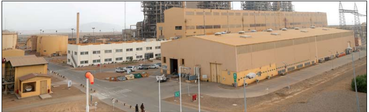
Hubco coal fired plant, Pakistan: NeuCo software is being delivered as part of GE's Digital Power Plant for Steam package
