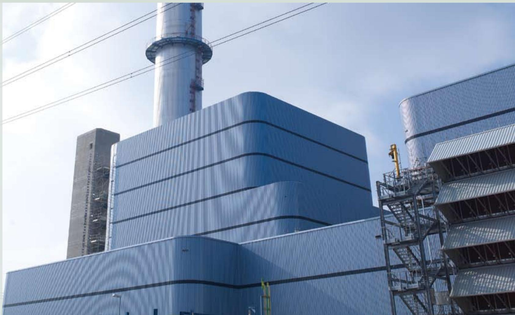
In 2011, E.On's Ulrich Hartmann plant in Irsching, Germany, became the first combined cycle power plant to break the 60 per cent barrier for electrical efficiency. It was also the first project to feature Siemens' 8000H advanced gas turbine.
