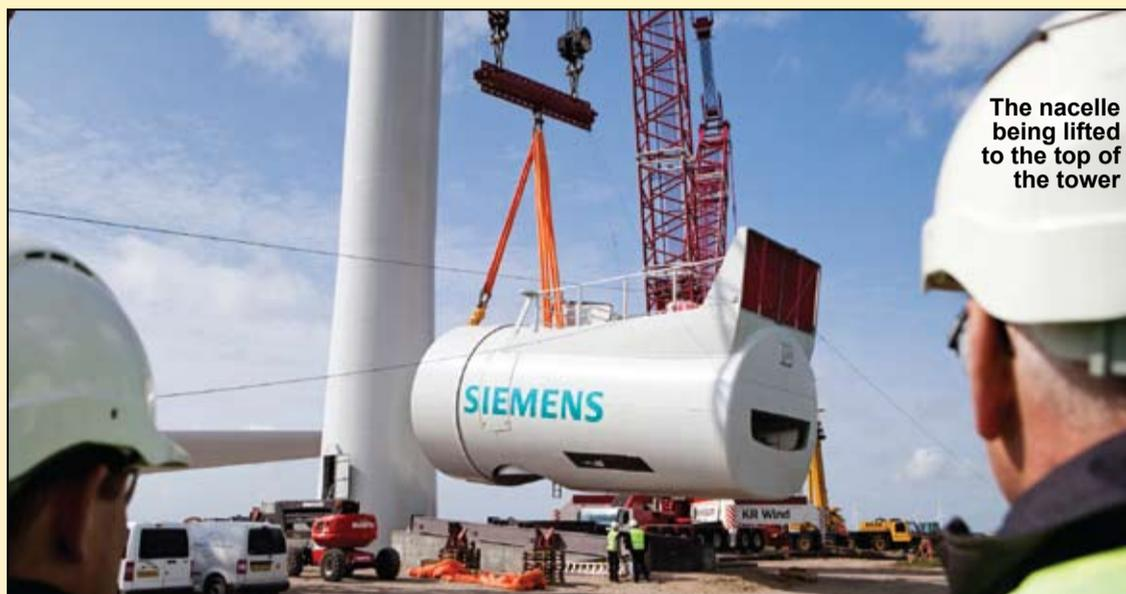
The nacelle being lifted to the top of the tower
