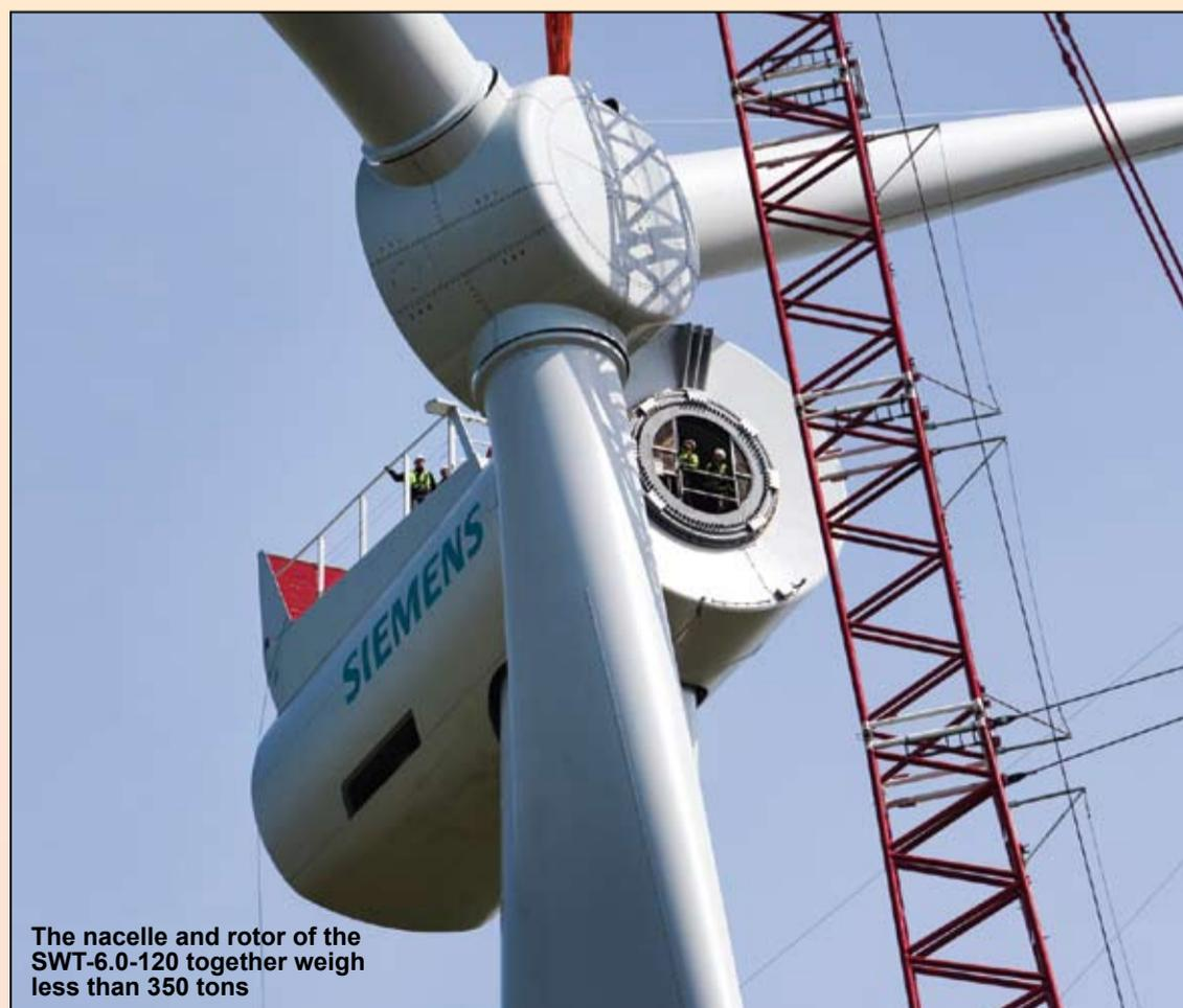
The nacelle and rotor of the SWT-6.0-120 together weigh less than 350 tons
