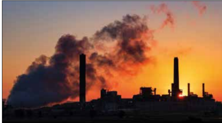
Topic of debate: Some operators are committing to low-carbon fossil fuel plant conversions to secure the future of installations
