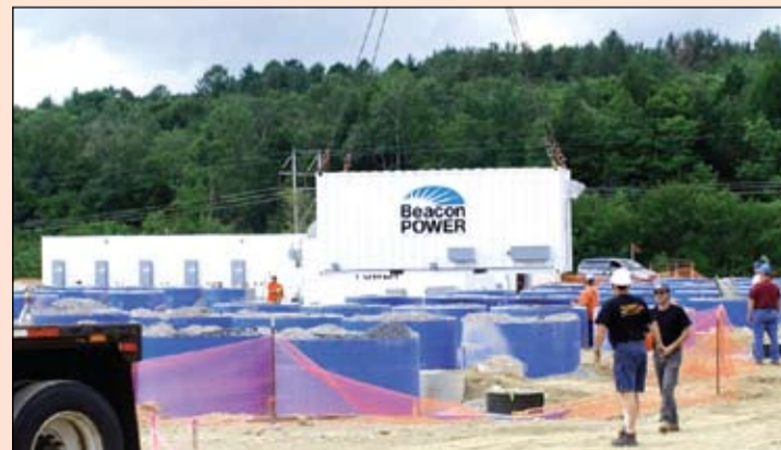
Beacon Power's pioneering flywheel energy storage plant
