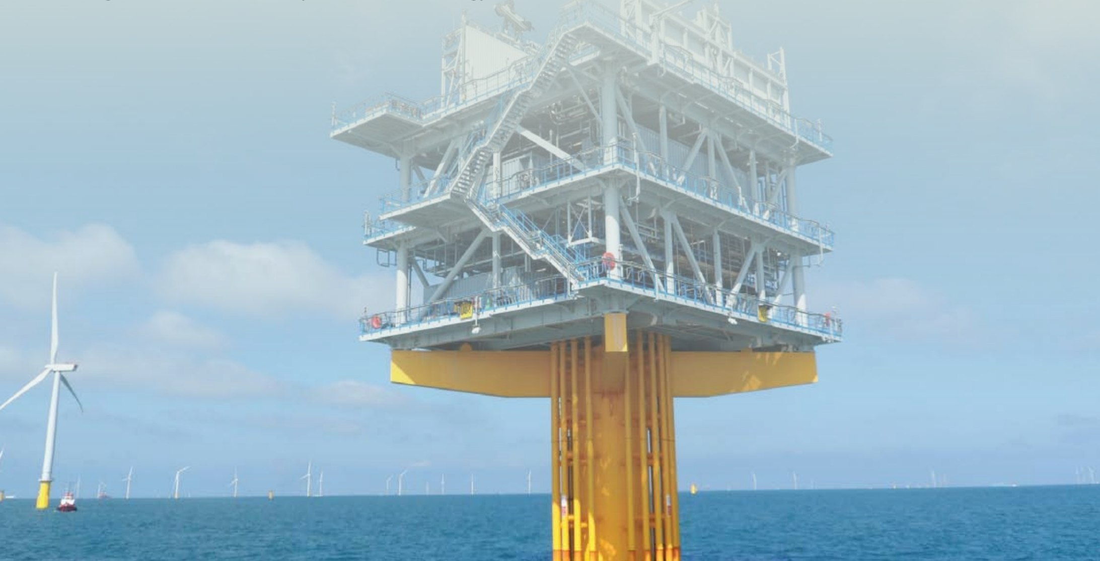
Turbines and substation at London Array. Copyright London Array Limited
