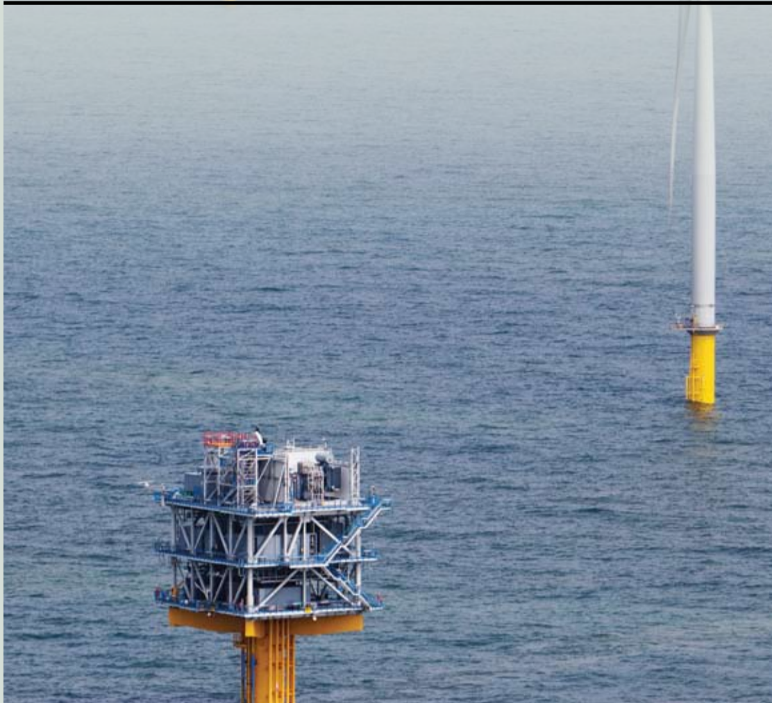
The London Array offshore wind farm where Siemens supplied the turbines and provided the grid connections
