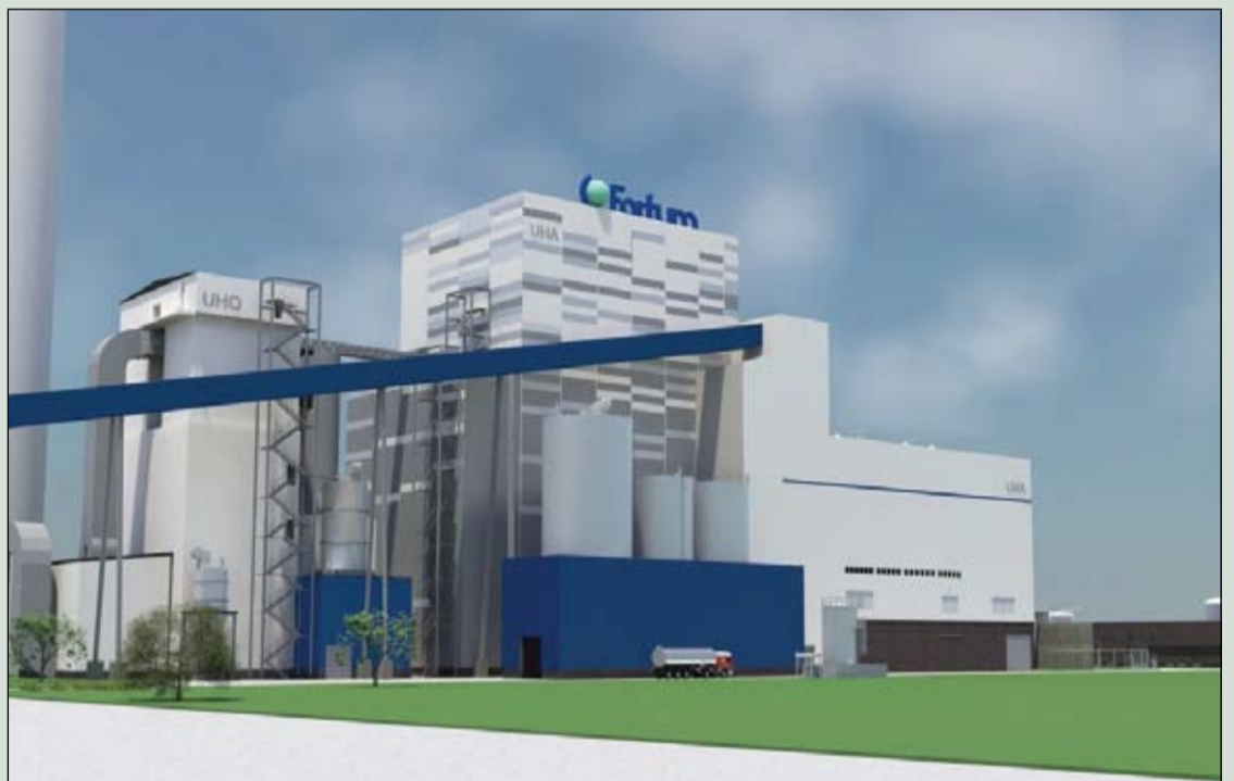
The Zabrze multi-fuel combined heat and power plant will begin commercial operation this year
