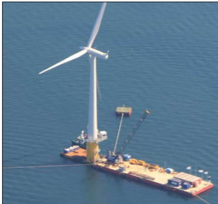
The 2.3 MW Hywind demonstration project being installed in 2009. © 2009 Jarle Vines
