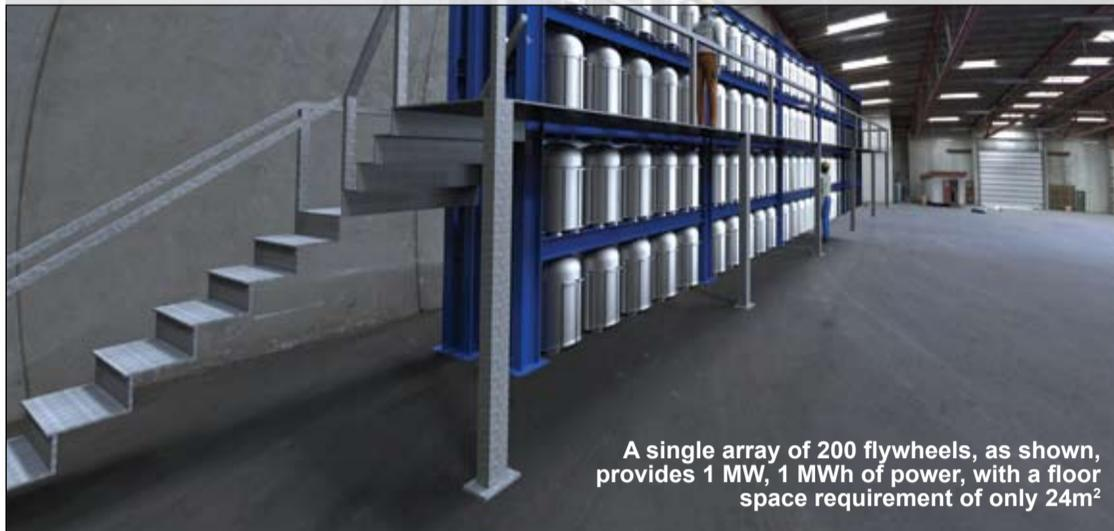
A single array of 200 flywheels, as shown, provides 1 MW, 1 MWh of power, with a floor space requirement of only 24m<sup>2</sup>
