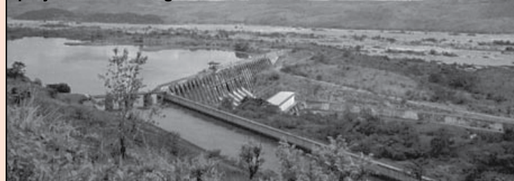
Revitalised: The 40 000 MW Grand Inga hydropower project on the Congo River
