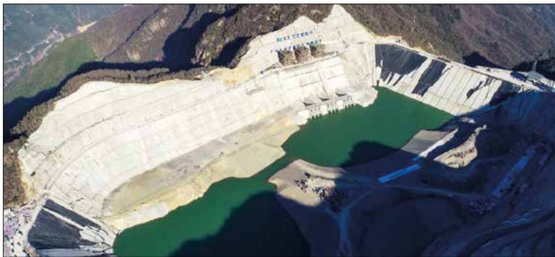
Bird's-eye view of the Changlongshan pumped storage hydropower plant
