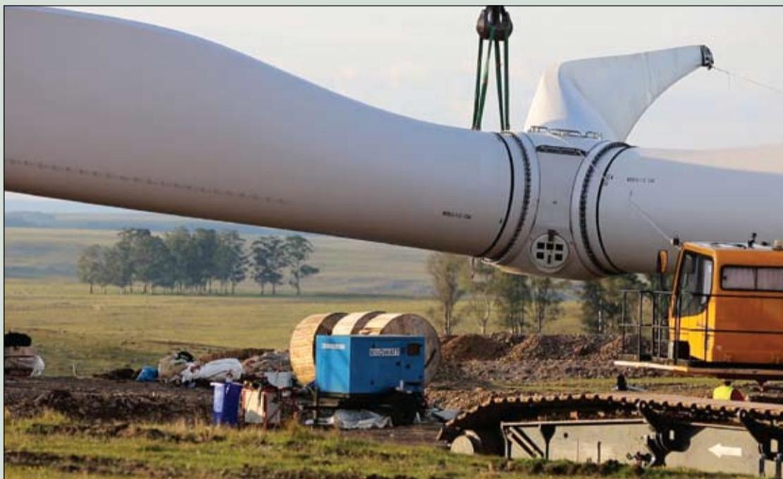
**Turbine blades were assembled on the ground before being "star-lifted" to the top of the tower**
