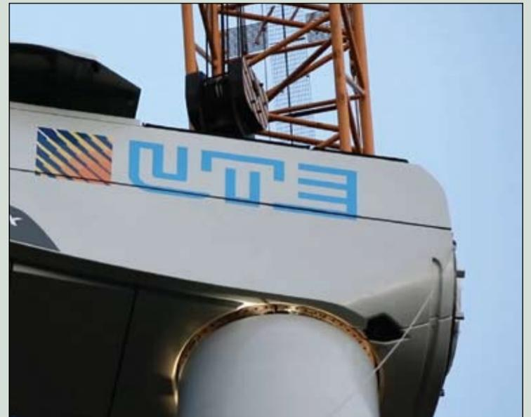
**A nacelle being installed at the top of a tower**
