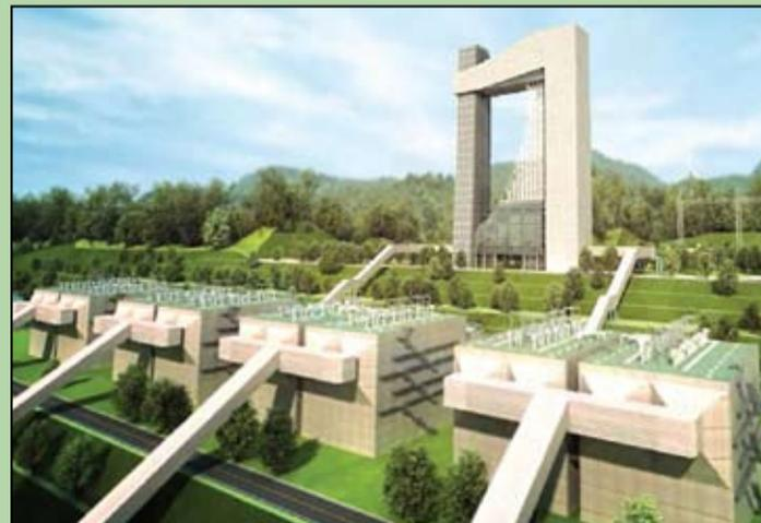
The coal units’ stacks are integrated with the office buildings in an architectural design
