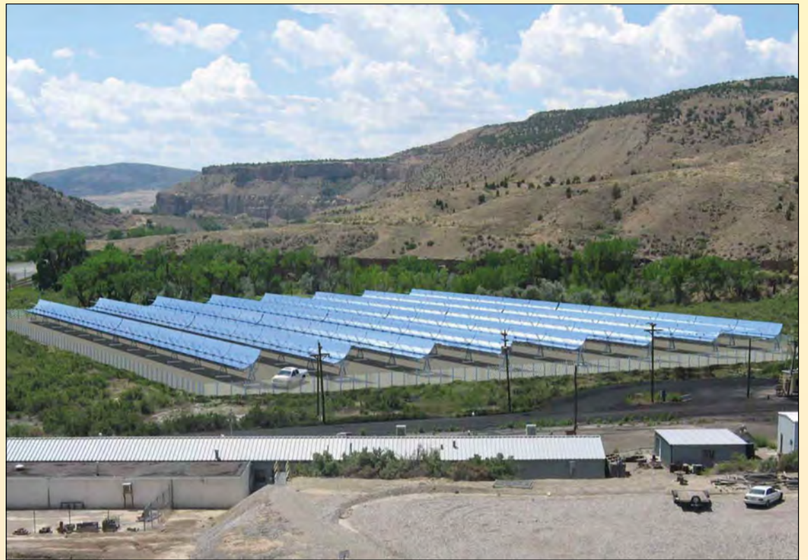
An artist's rendering of the CSP installation at Cameo. It will be operated for approximately a year to evaluate the CSP technology and its impact on the coal plant
