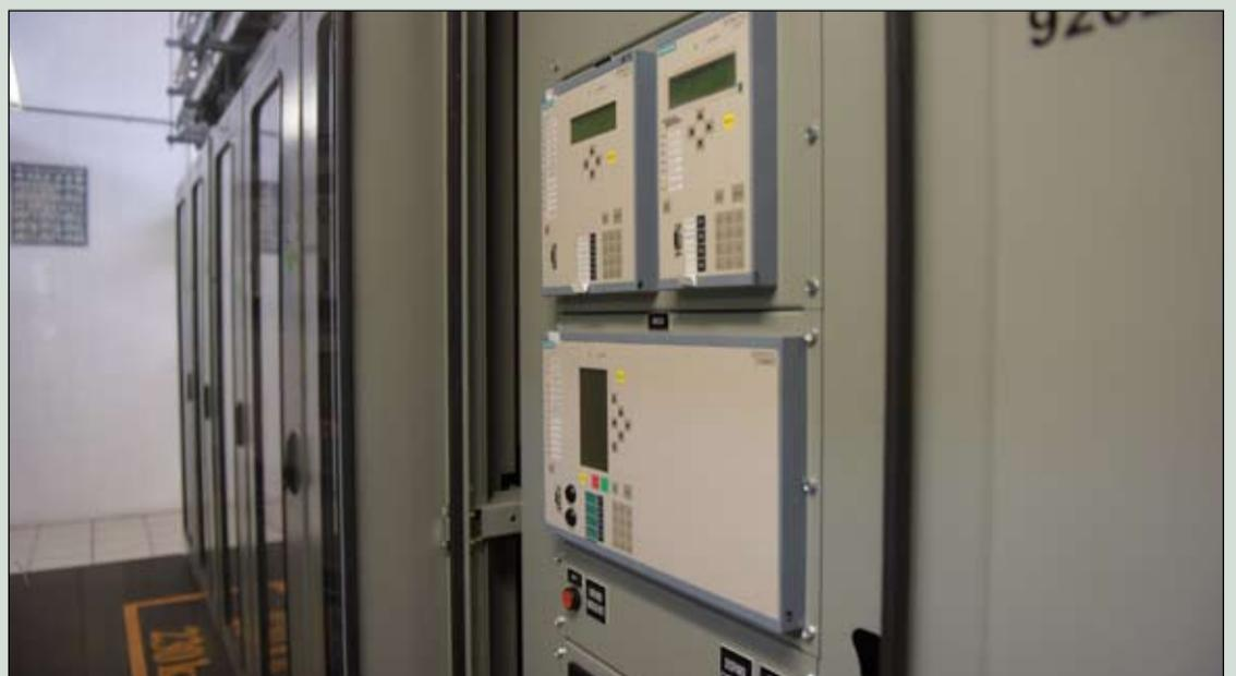
**Protection, control and measurement cabinet inside the substation at the Buenavista del Cobre mine**
