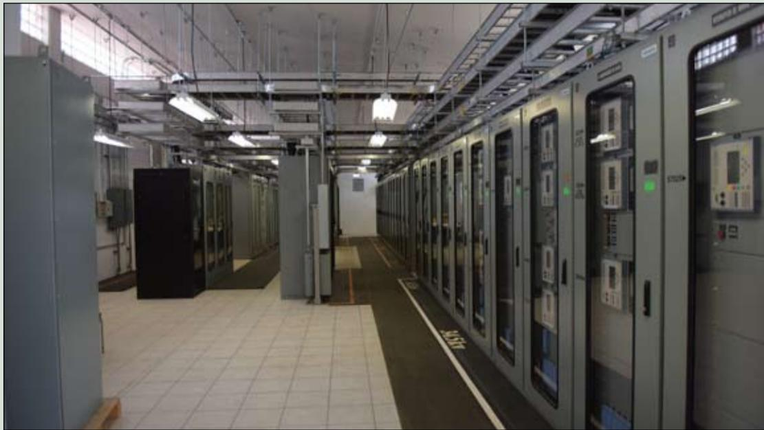
**Substation main protection, control and measurement room. The new network control system has seen a 60 per cent reduction in downtime**
