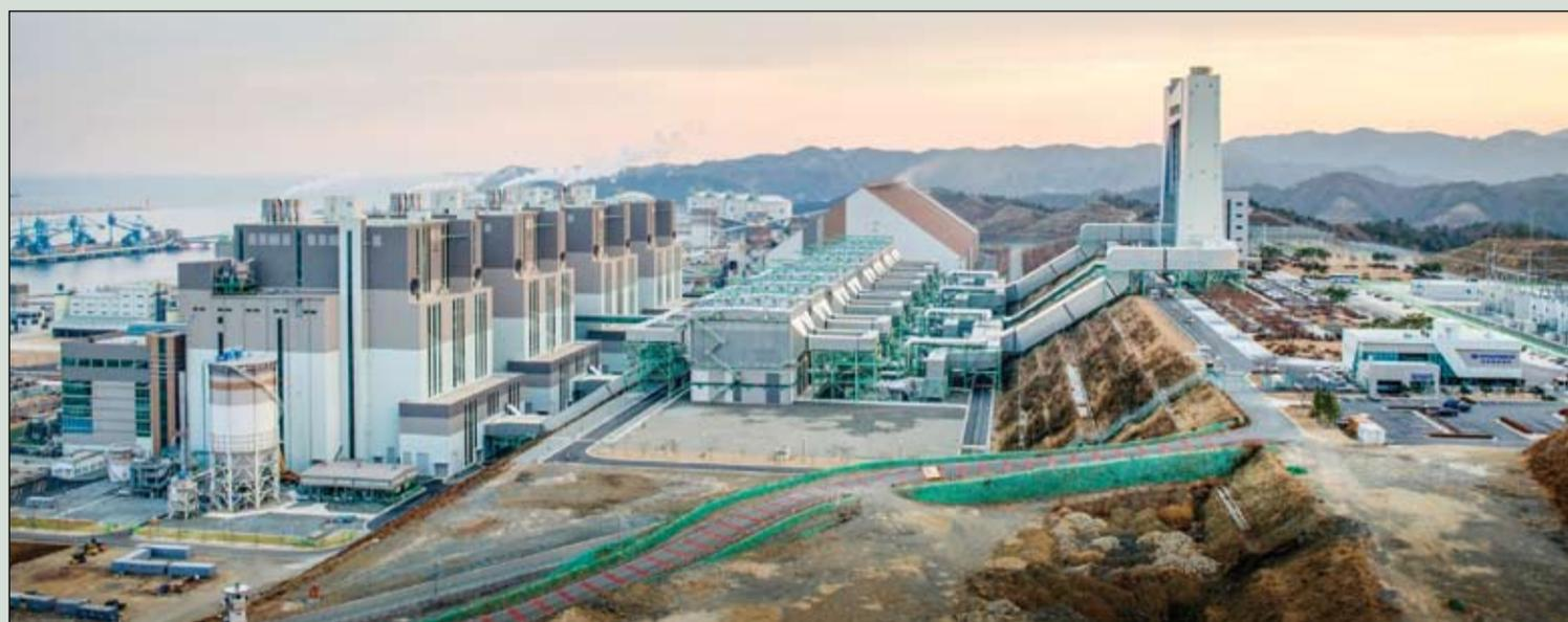
took place on February 29, 2016 followed by boiler 1A a few weeks later. Commissioning activities continued with magnetite film formation, curing of the refractory linings and steam blowout process as a final step before the start of boiler testing and the tuning period.
