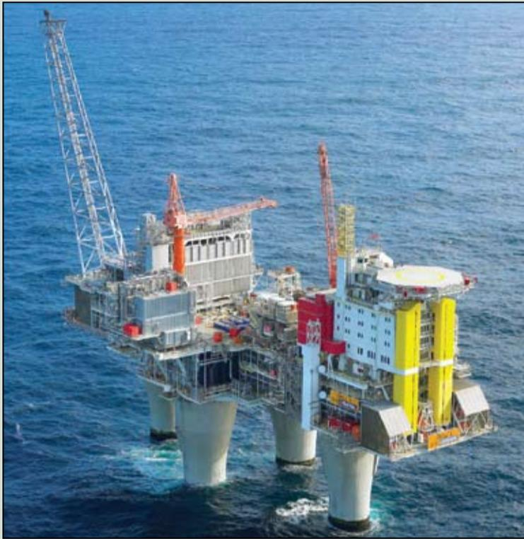
**The Troll A platform was the world's first offshore transmission using HVDC Light technology**
