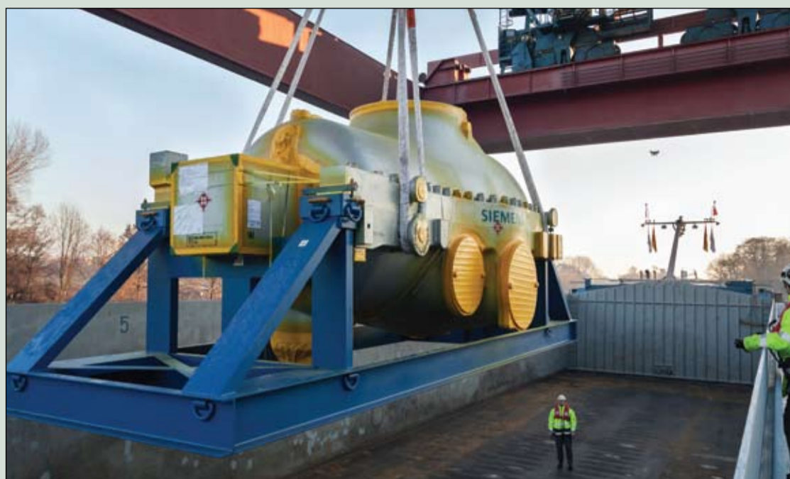
Steam turbine components being lifted on to the transport vessel. The first steam turbine arrived at North Sea port in December 2016
