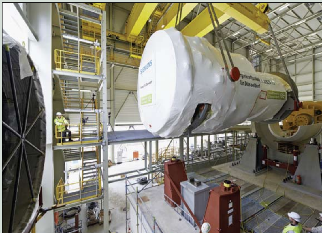
Installation of the SGT5-8000H gas turbine at Fortuna
