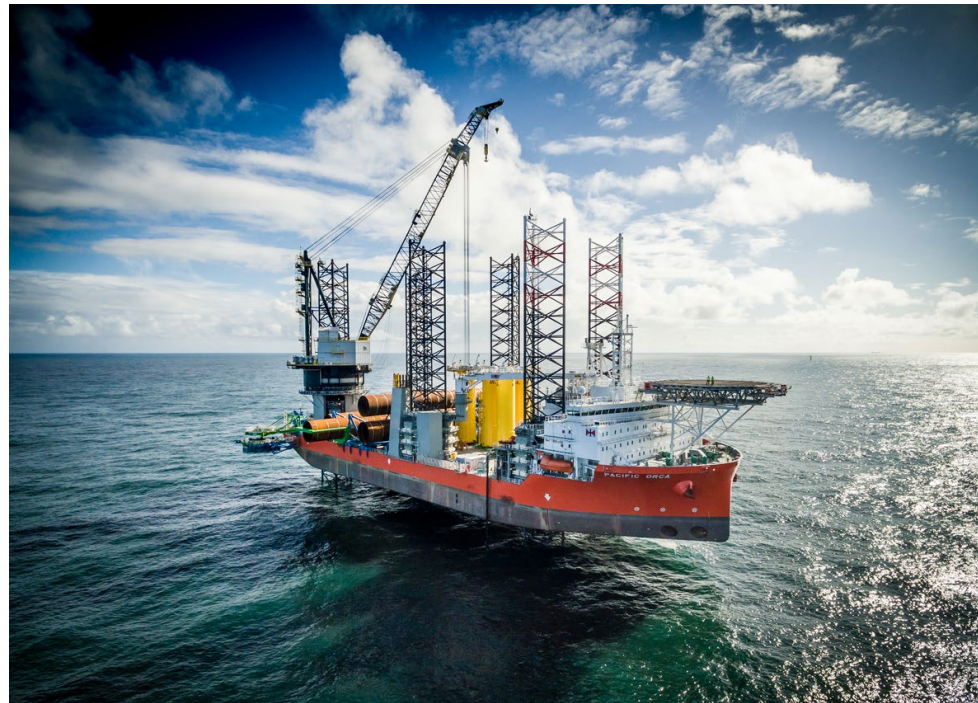
VATTENFALL'S SANDBANK OFFSHORE WIND FARM IN THE GERMAN NORTH SEA. SOURCE: VATTENFALL
