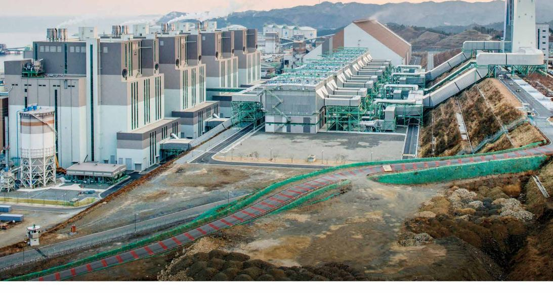
The massive 2.2 GWe Samcheok Green Power Projectin South Korea is approaching two years of full commercial operation. Utilizing the most advanced ultra-supercritical CFBs in the world, it signifies the next big step for clean and flexible power from economical solid fuels.
