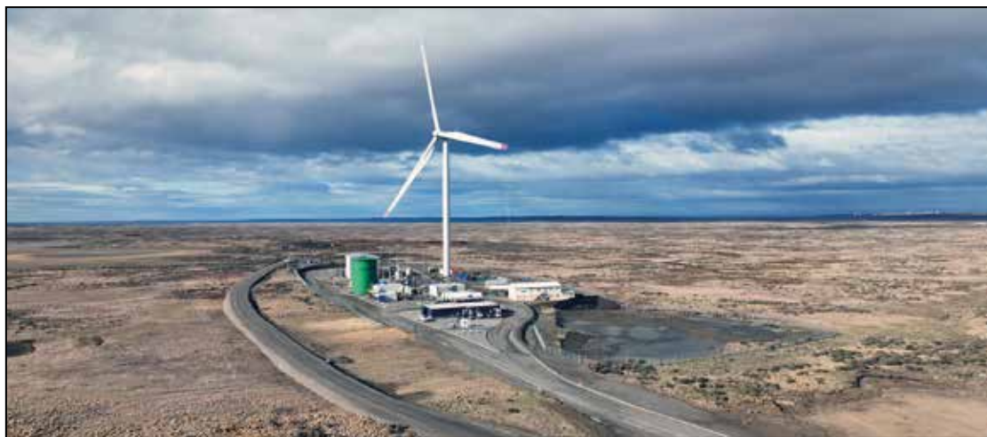
The Haru Oni project uses wind power to produce hydrogen and direct air captured CO 2 to make e-methanol in a reactor from MAN Energy Solutions
