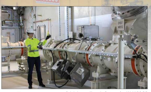
sits at the heart of the project. The platform utilises Siemens Energy's HVDC Plus technology to convert power from AC to DC. It is based around the Modular Multi-level Converter (MMC) for high voltage, high power voltage source converter (VSC) applications.
