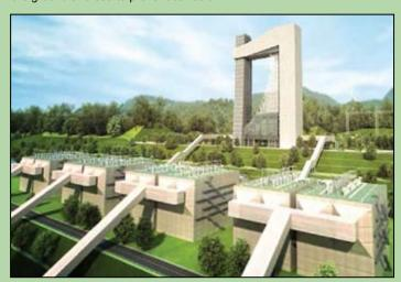
The coal units' stacks are integrated with the office buildings in an architectural design
