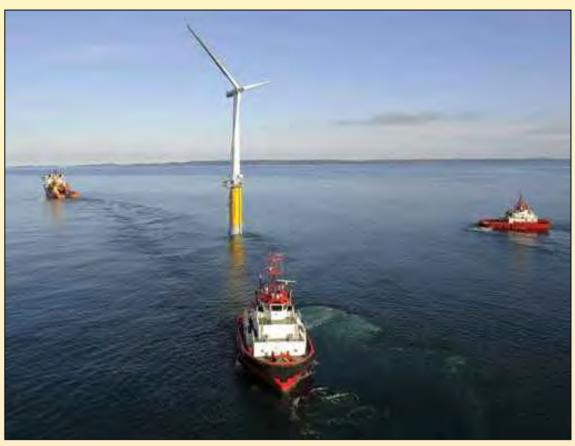
The world's first large-scale floating wind turbine is located approximately 10 km south east of Karmøy in Norway at a water depth of about 220 m
