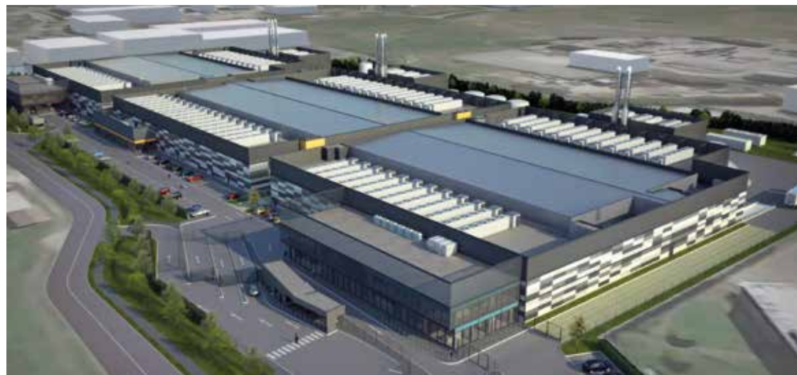
Artist impression of the data centre near Dublin, where construction is well underway
